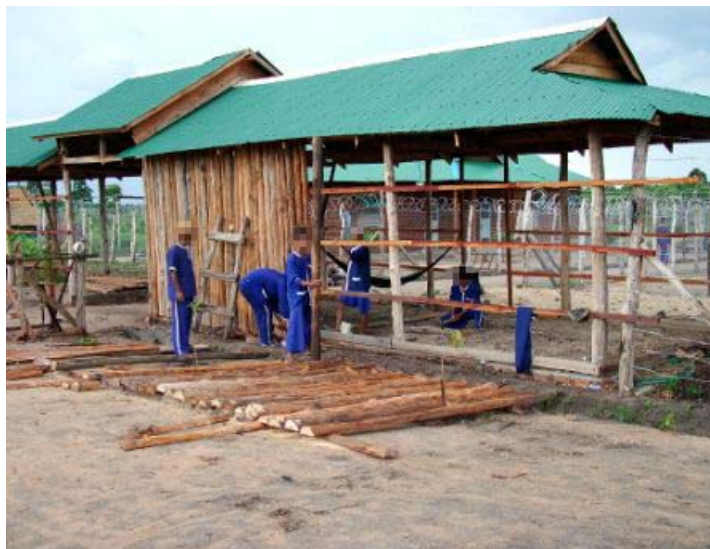
Inmates labor is being used to construct CC4. (Photo Supplied)
